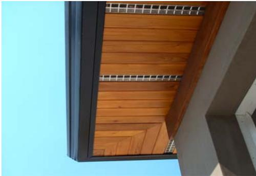
Vents are important for the healthy air exchange and moisture escape required in a building. They also are ready-made accesses into a building. Unprotected eaves can allow burning embers to enter and also allow flames that are spreading up a wall to penetrate into the roof structure.
