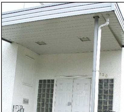
As with roofs, decks present a large horizontal surface for burning embers to land on and take hold. In addition, decks have an underside that can trap embers and be a source of fuel for fires. It is important to enclose the underside of decks and large overhangs.
