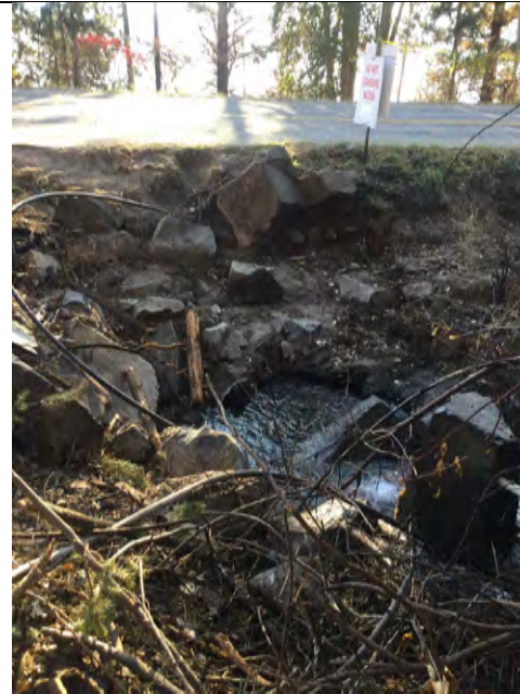
Photo 10: Lower Luluwap Creek crossing at Westside Road (damaged 600 mm culvert) (Lower Luluwap-1)
