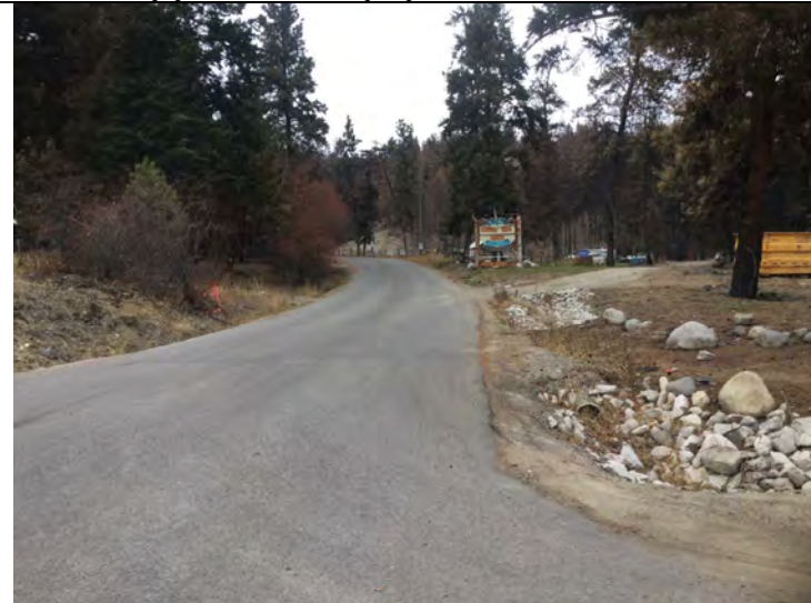
Photo 12: View of ditch line along Petterson Road (at Bear Creek Road), conveys surface water runoff from Upper Luluwap Creek area.
