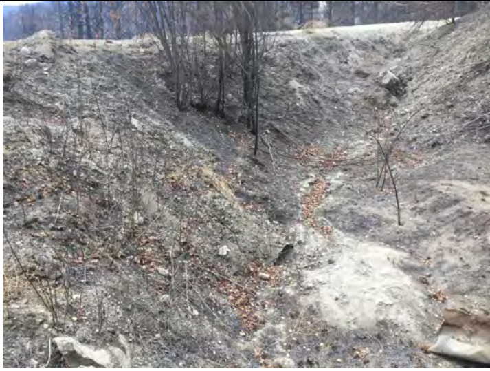
Photo 8: Mostly plugged culvert inlet on upslope side of Bear Lake Main FSR at Blue Grouse Creek crossing (Blue Grouse-1)
