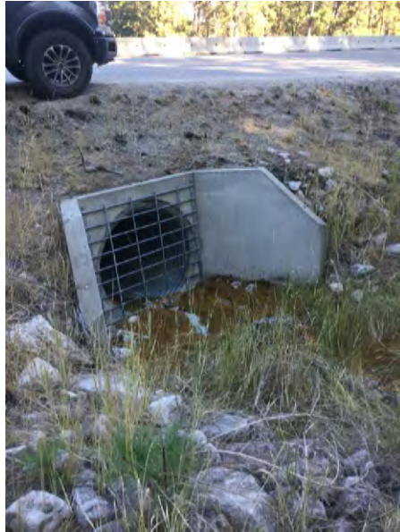
Photo 3: New 1200 mm culvert with trash rack and rock lined channel on Dimetri Creek at Westside Road (Dimetri-1)
