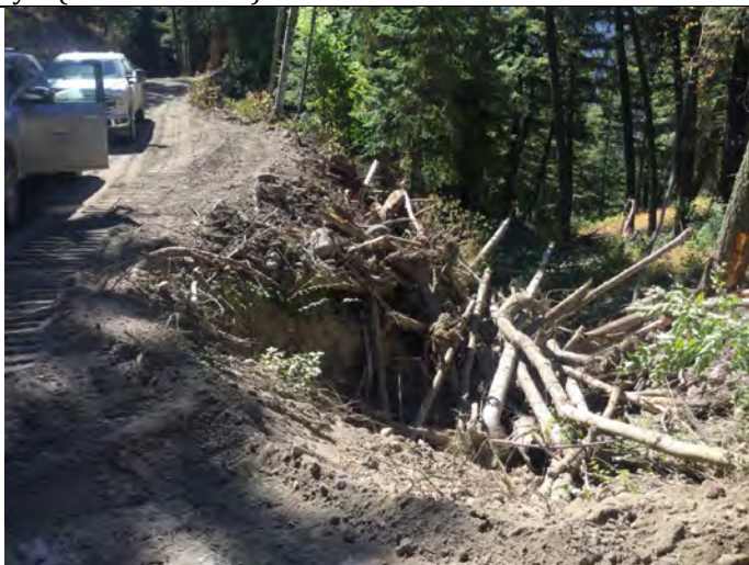
Photo 3: Road crossing (due to be rehabilitated) on Powers Creek Tributary 1 with abundant sediment and woody debris (Powers-Trib-2)
