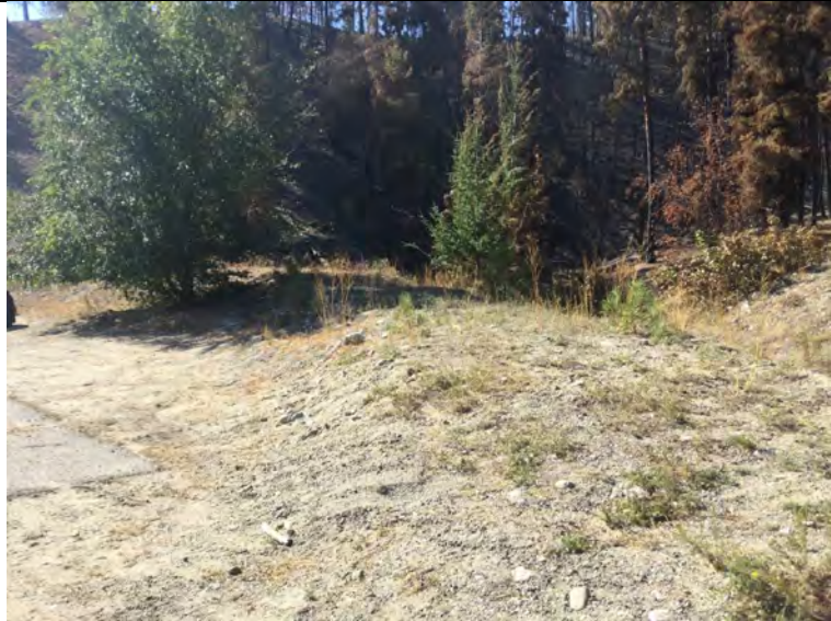
Photo 11: Shallow, discontinuous berm along upslope edge of Fire Hall Parking lot (Wilson-1)
