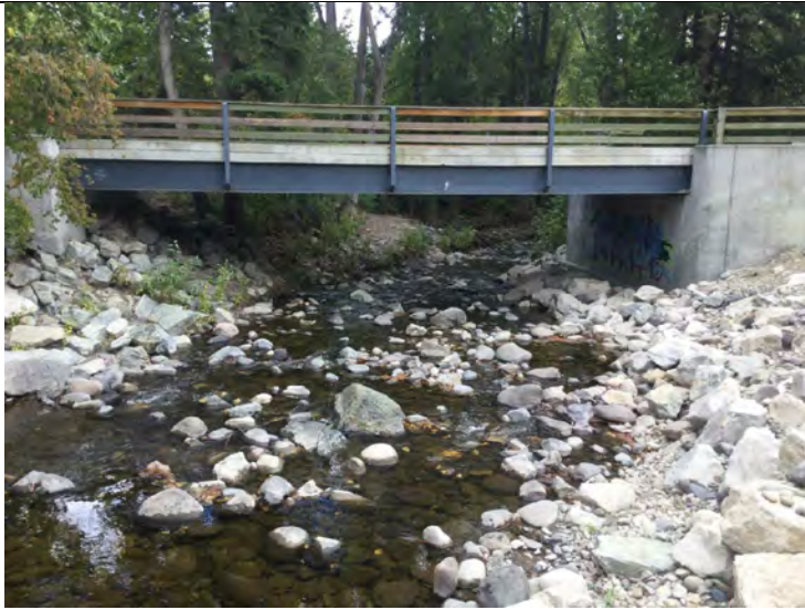
Photo 1: Lambly Creek bridge crossing within the Bear Creek Provincial Park Campground, showing good clearance (Lambly-1).
