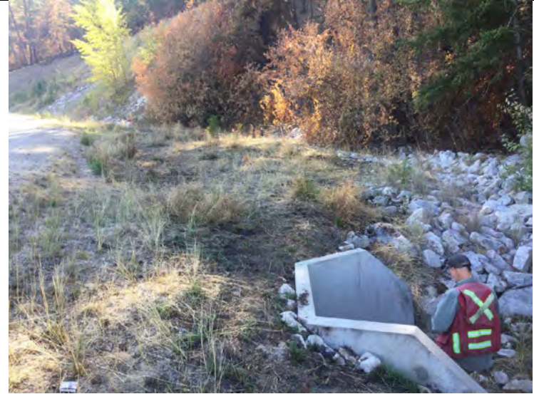
Photo 2: New 900 mm culvert with concrete baffles and rock armour on Cinnabar Creek crossing Westside Road (Cinnabar-1).
