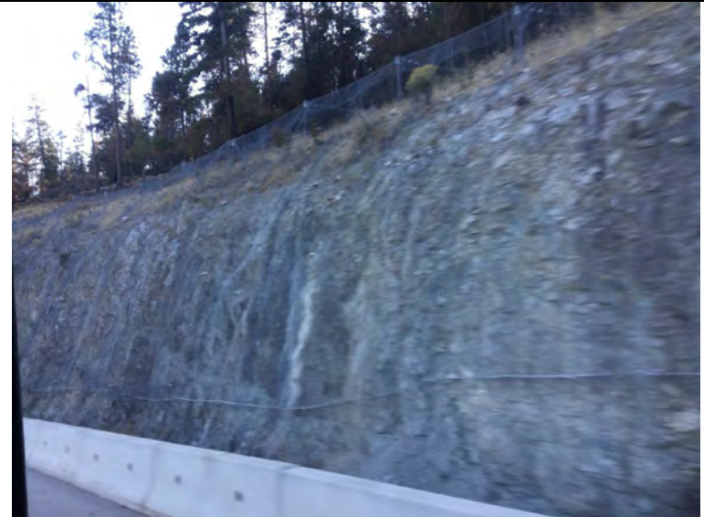
Photo 20: Rock cut with rockfall protection fencing along Westside Road.
