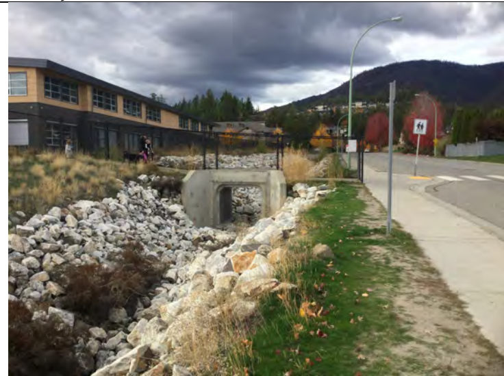
Photo 4: Rock-lined channel and concrete culverts on Faulkner Creek in front of Mar Jok Elementary School (Faulkner-4).
