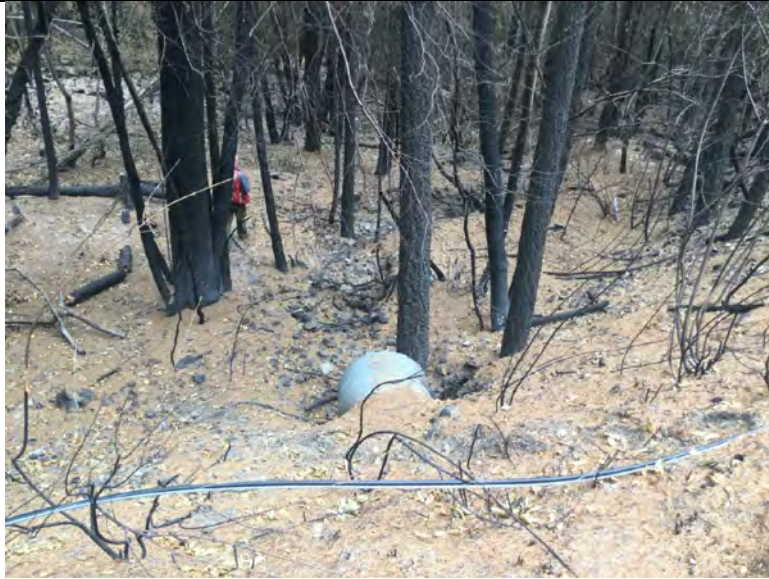
Photo 28: View downstream from Bear Creek Road at culvert crossing. Note abundant colluvium, and hummocky terrain indicative of past flood events. (Cedar-4)
