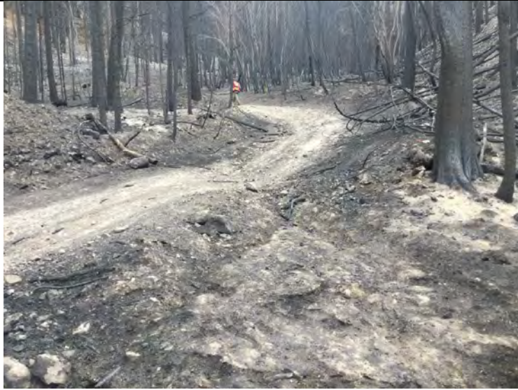
Photo 9: High vegetation burn severity area, with observed sediment-laden runoff along road and variable soil-water repellency (McDougall-6)
