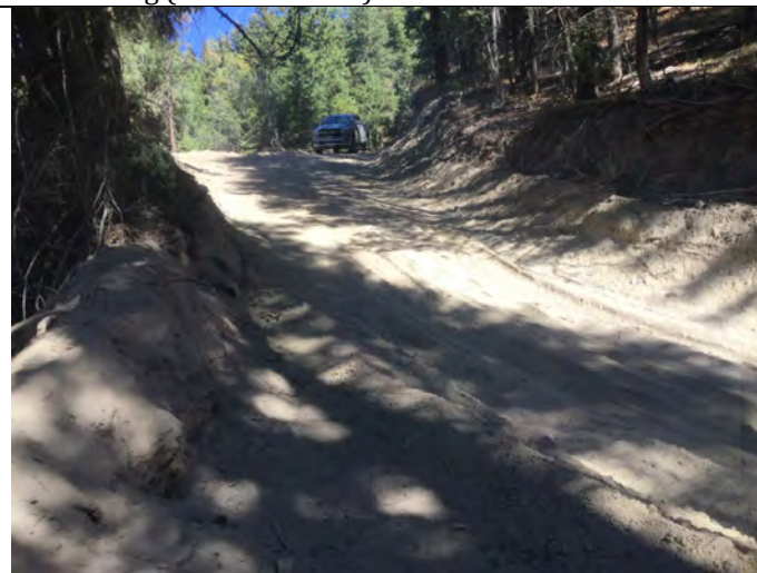
Photo 4: Downcutting of fine-textured silty sediments along road used to access the fire (downslope of Powers-Trib-2)
