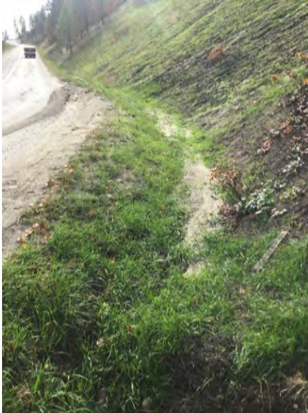
Photo 7: Sediment-filled ditchline along Bear Creek Road, at Westside Road (Keefe-3)
