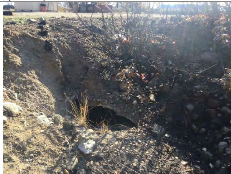
Photo16: Inlet of 1000 mm culvert on Jennie Creek at Westside Road is mostly blocked with sediment (Jennie-1)
