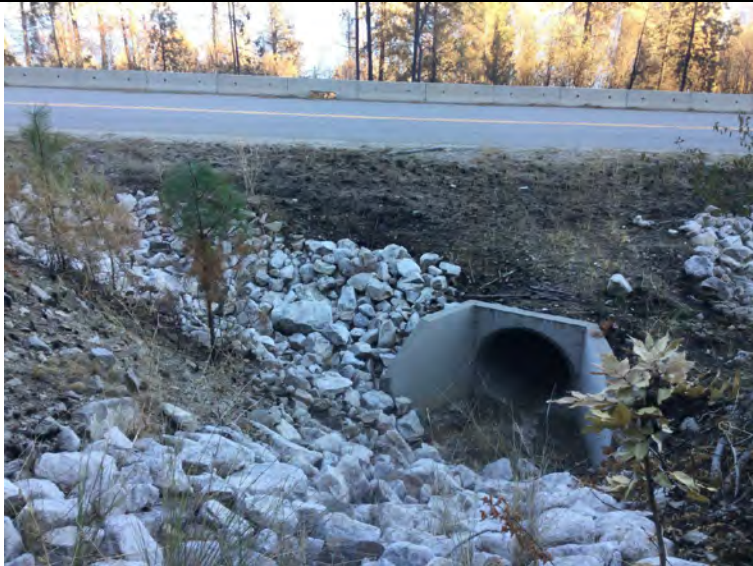
Photo 19: Newer 1200 mm culvert with concrete baffle and rock-lined ditch along Westside Road.
