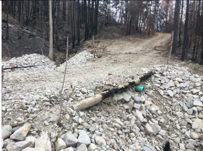
Photo 22: Cedar Creek crossing at Water Pipeline (500 mm plastic pipe and 200 mm plastic pipe). Note, burned log stringers. (Cedar-1)
