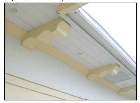
Vents are important for the healthy air exchange and moisture escape required in a building. They also are ready-made accesses into a building. Unprotected eaves can allow burning embers to enter and also allow flames that are spreading up a wall to penetrate into the roof structure.
