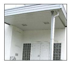
As with roofs, decks present a large horizontal surface for burning embers to land on and take hold. In addition, decks have an undersurface that can trap embers and be a source of fuel for fires. It is important to enclose the underside of decks and large overhangs.
