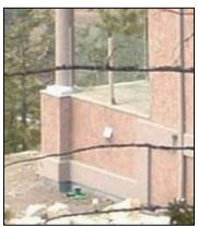
Remember that open frame construction can trap burning embers that not only fall from above but also are blown in from all directions.
