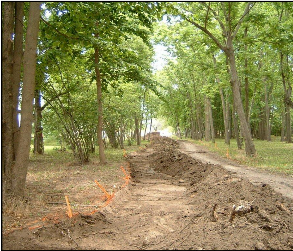
Figure 23. Access road construction caused root damage to the adjacent trees (RDCO, 2005).
