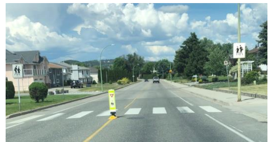
Figure 38. Installation of in-street school crosswalk sign
