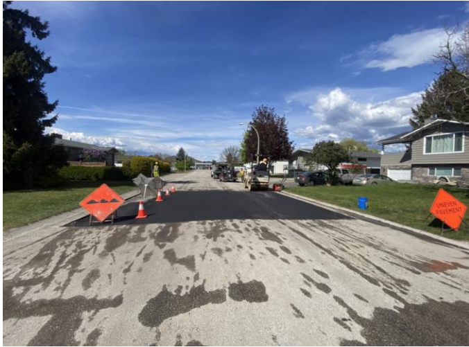
Figure 49. Collison Rd speed hump construction
