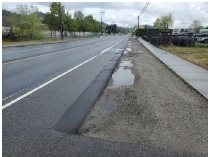
Figure 35. Ziprick Rd asphalt fillet to widen bike lanes and maintain parking
