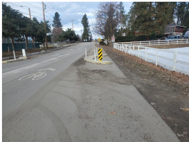
Figure 28. Traffic calming curbs and sharrows- Spiers fronting SKE north of parking lot access
