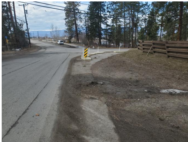
Figure 27. Traffic calming curbs- Spiers & June Springs
