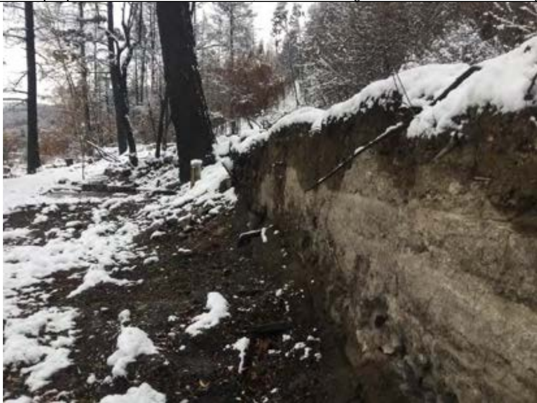
Photo 2: Close up view of burned wood retaining wall at 55 Killarney Pl.
