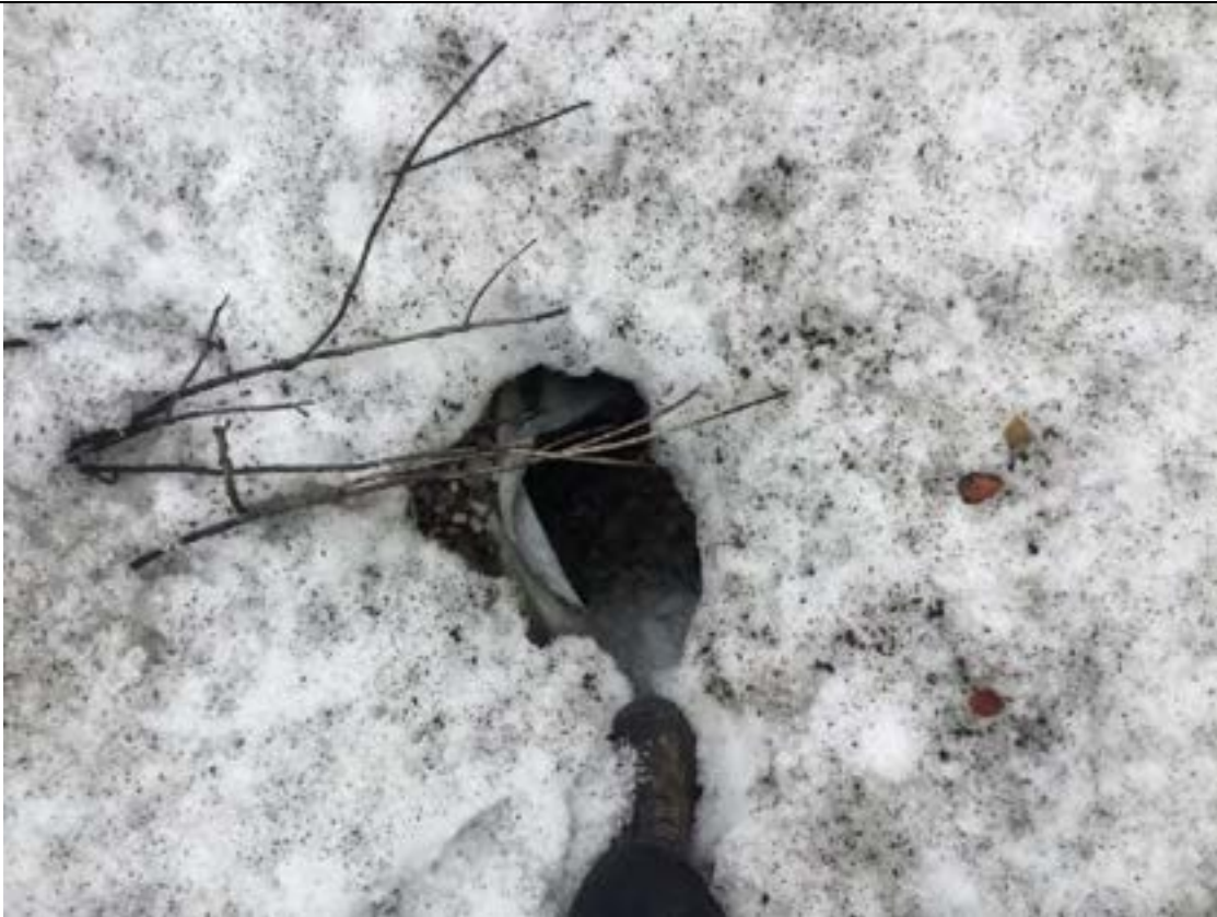
Photo 3: Partly obscured inlet of ~400 mm culvert at 8700 N Westside Rd.
