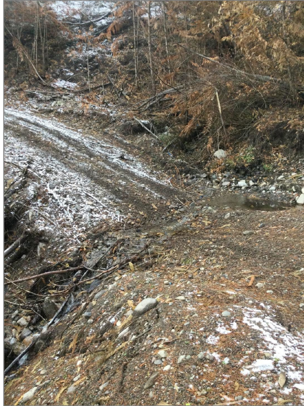
Figure 4-3: Unstable Fills at Trail Crossing on Norris Creek
