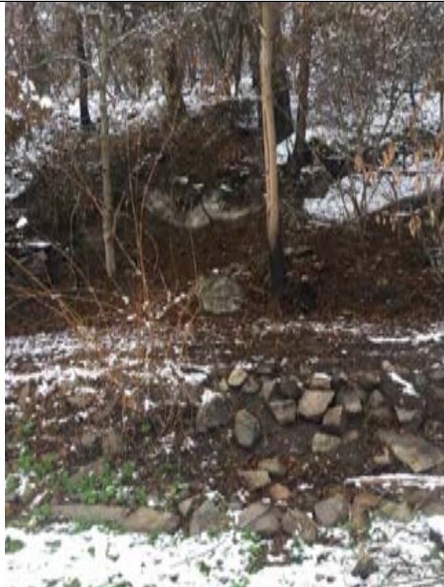
Photo 2: View of slope above foreshore area with rock retaining wall and driveway access trail above.
