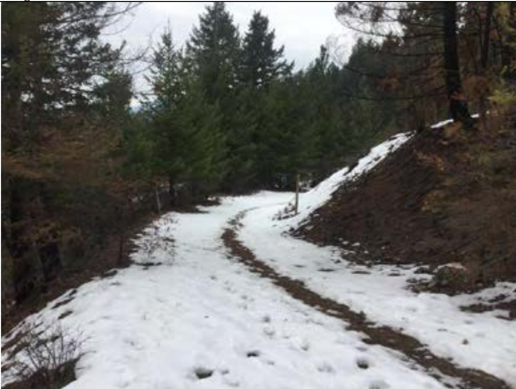
Photo 4: Unpaved access trail switchbacks off end of Killarney Pl. Minor raveling cutslopes and minor erosion along trail surface.
