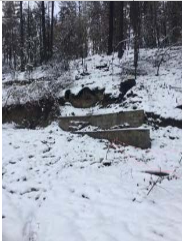
Photo 2: View of slope above foreshore area with block retaining wall along toe of slope
