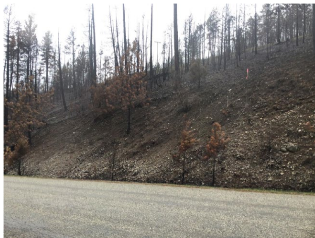
Exposed mineral soils above Beachwood Rd subject to soil erosion and shallow landslide
