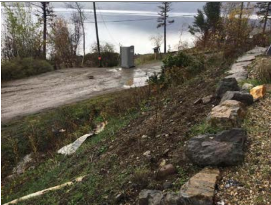
Photo 1: View of corner property at 104 Elliot Rd towards ditchline and culvert across Nerie Rd. Noted, two white PVC drain pipes along cutslope.
