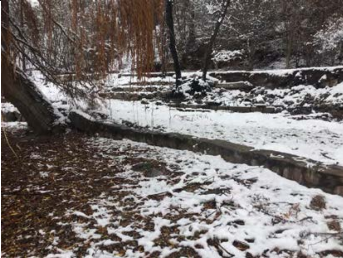
Photo 1: View upslope of foreshore area from the lake, concrete retaining wall and burned wood retaining wall
