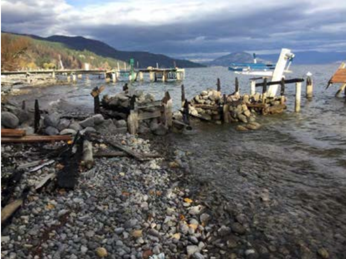
Photo 3: View of damaged dock with rock filled piling at 2 Nerie Rd.
