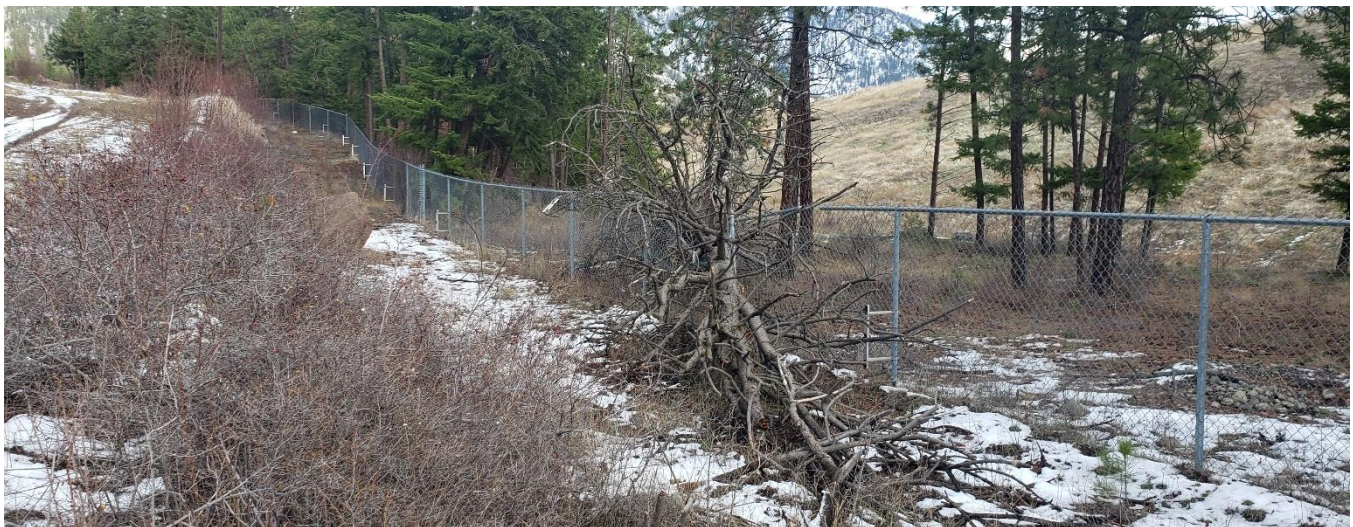
Photo 1: Damaged perimeter fencing along western property boundary due to fallen tree, facing northeast.
